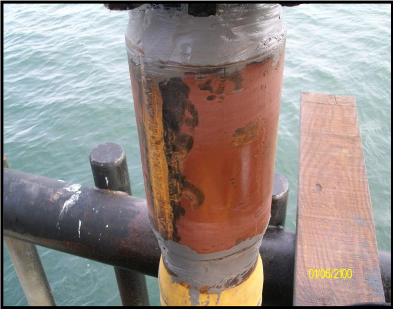
6" Before RiserWrap™ Installation.
