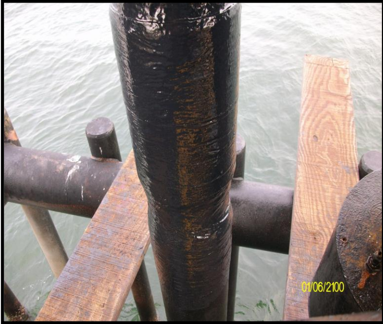
After RiserWrap™ Installation
