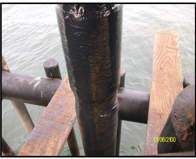
Second View 6" RiserWrap™ Installation.
