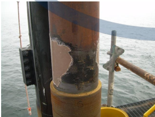
Completed Molding Process
