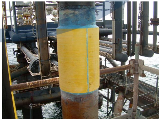
Completed Clock Spring Installation
