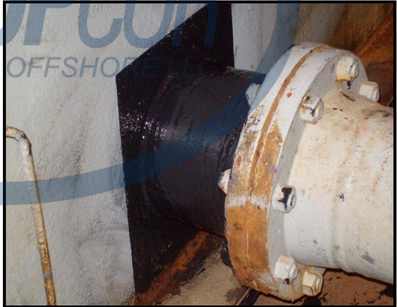
Completed RiserWrap Installation over Repair Area.
