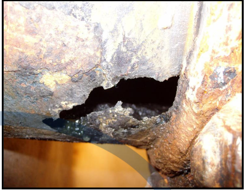
After Surface Preparation
