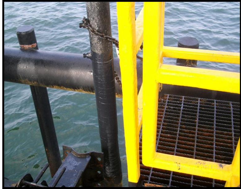
4" Riser after RiserWrap Installation.
