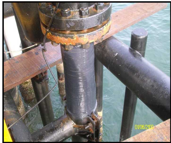
4" Riser after RiserWrap Installation.
