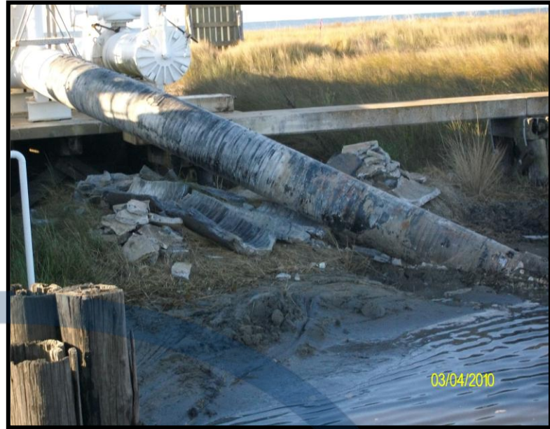
Concrete Removed
