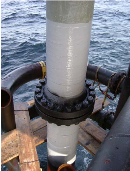
Corrosion Inhibitor Applied to Flange
