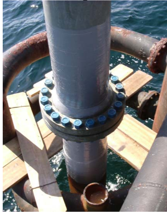
RiserWrap ™ Applied as Corrosion Barrier
